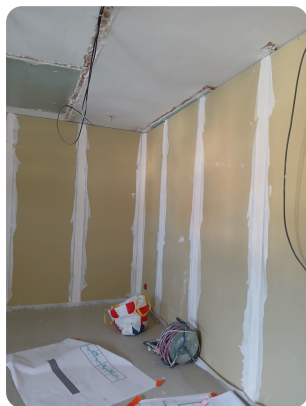
joints de cloisons
